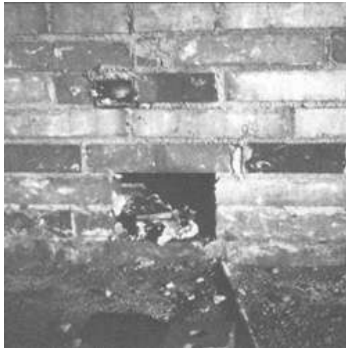
Grout Cleanouts Fig. 17
