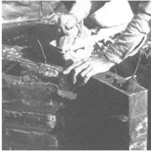
Sponges In Cells To Be Grouted Fig. 16
