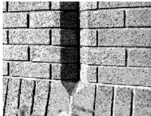
accentuated Vertical Expansion Joint
