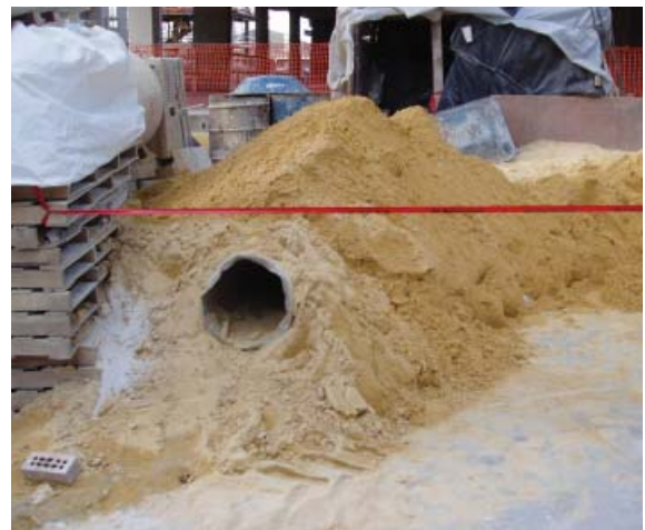
Photo 3 Sand Pile Warmed by Heated Pipe
