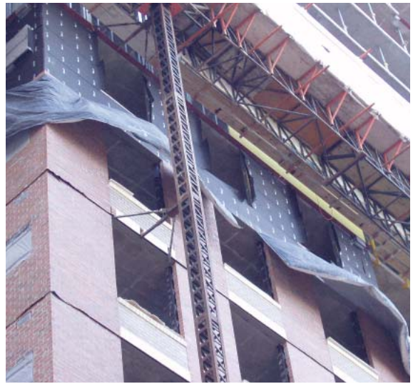
Photo 1 Cover Protecting Newly Constructed Masonry
