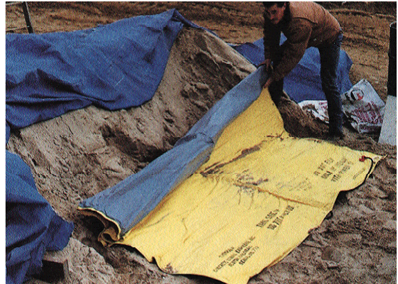
Photo 2 Heating of a Sand Pile with an Electric Blanket
